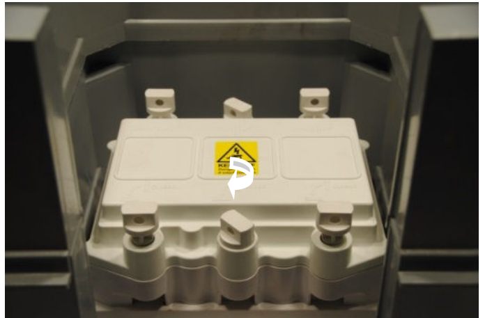
4. Turn opposite centre toggle an 1/8" of a turn as shown
