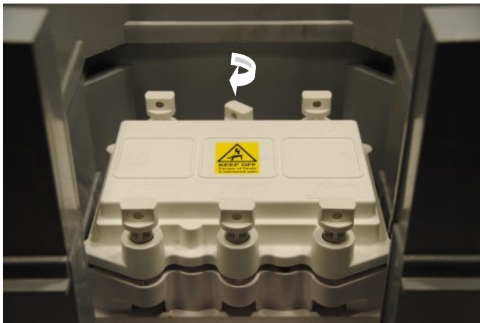
3. Turn Centre toggle 1/8" of a turn as shown
