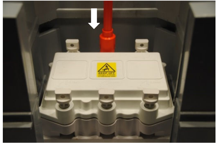
2. Using recommended tool depress centre toggle
