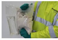
2. Aerate the powder by gripping the pouch at each end and tumbling the powder for up to thirty seconds, this will facilitate mixing
