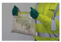
3. To start the mixing process, hold the bag as shown above, so that the liquid is forced onto the powder.
