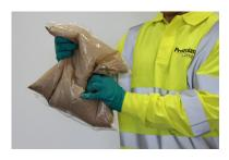
7. Tumble mix and knead the bag for up to two minutes, to ensure that there are no lumps in the bag.
