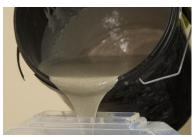
8. Pour fully mixed resin from the bucket into the joint shell.
