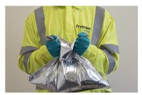
3. Squeeze the hardener through the membrane into the resin (large) compartment.
