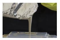
8. Pour pouch contents into the joint shell.
